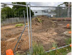
A layer of low quality soil (sand, clay) will be topped with good quality top soil and grass planted. The oval is raised higher than previously with underground drainage channels and a slight northerly slope to improve drainage after heavy downpours.
