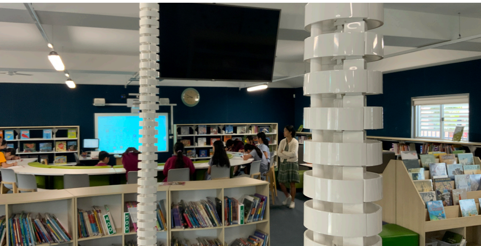
UMBILICALS WITH ELECTRICAL CABLES ALLOW THE RETURN'S DESK TO BE LOCATED IN THE MIDDLE OF THE LIBRARY
