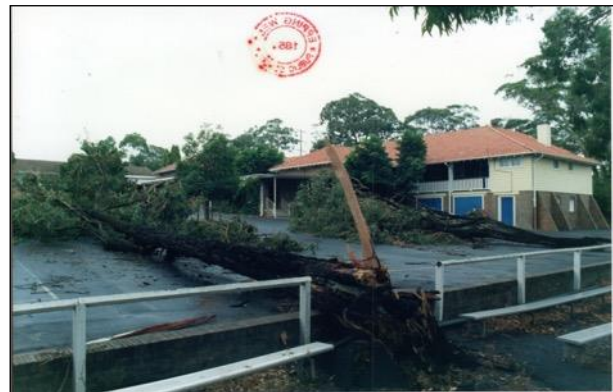
Storm Damage at the school January 1991
